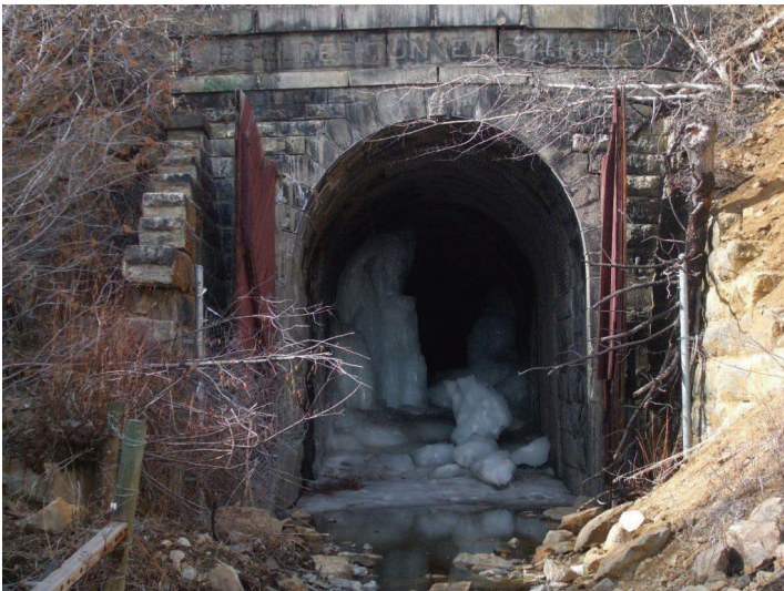
The Great Northern's Boulder Tunnel
