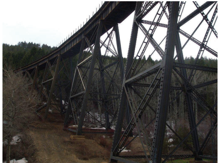
Montana Rail Link's Austin Creek Trestle
