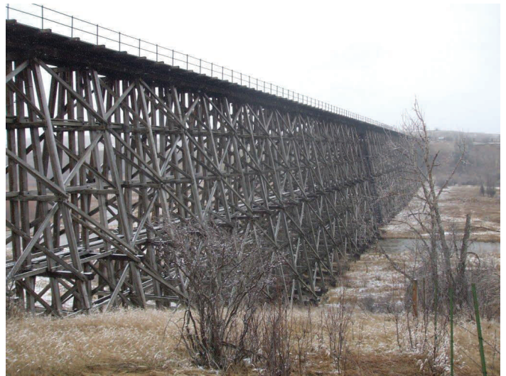
Milwaukee Road's Spring Creek Trestle
